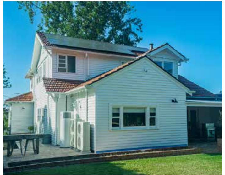
Solar panels complete the electrification of this home in outer East Melbourne
